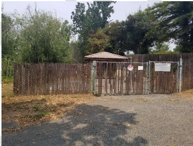
Photo 3 Lift Station 1 Site
