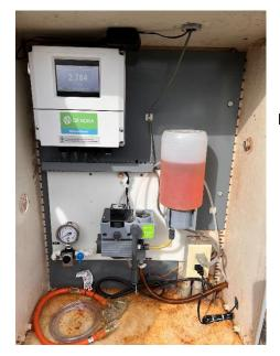
New chlorine analyzer at the end of the CL2 contact basin.
