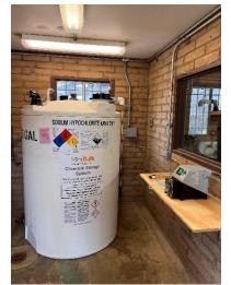
Chlorine room 405 gallon 12.5% CL2 storage tank and chemical feed pump.
